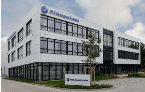
Headquarter of HS Elektronik Systems GmbH in Nördlingen, Germany
