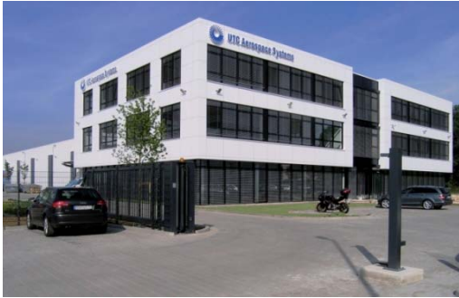
Headquarter of HS Electronic Systems GmbH in Nördlingen, Germany
